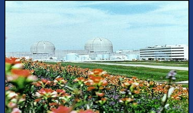
South Texas Project
