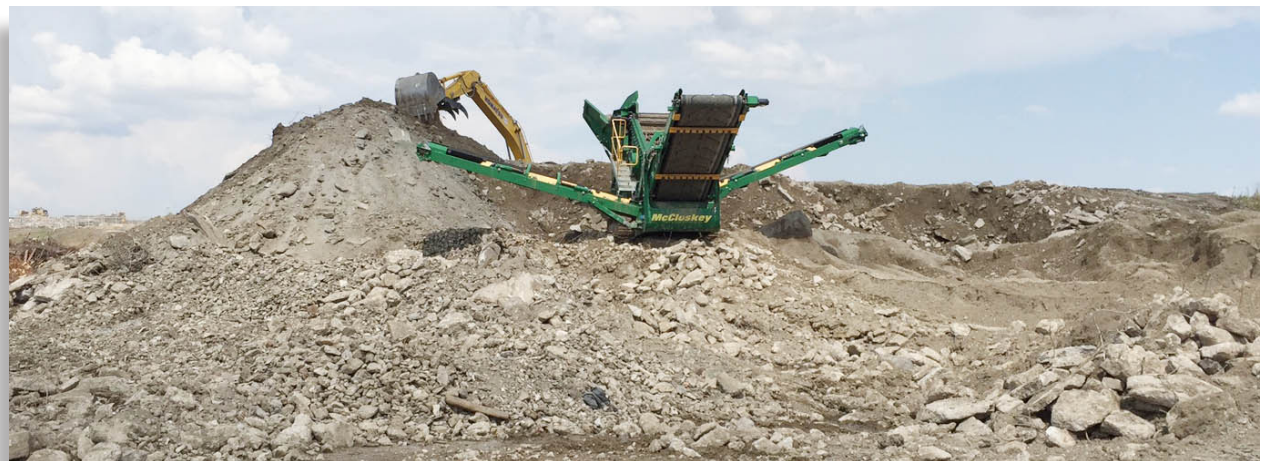
The City processes concrete into flex-base material, with the remainder being used to fortify the perimeter road at the landfill.
