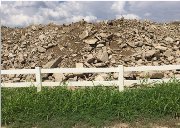
A landfill accepted construction and demolition waste in the form of a concrete/soil composite which had been stockpiled and periodically ground on-site by a local vendor.
