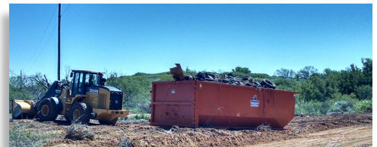
The project allowed the County to rent an excavator and roll-off containers to remove the materials for sorting. The County cleaned up 19,140 pounds of waste.
